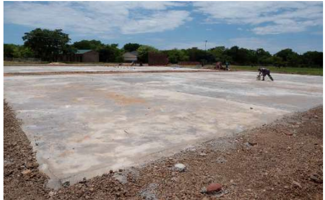
New sports facilities being constructed
