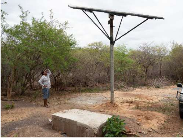
The new borehole – the pump is enclosed in very thick concrete. Security cameras are being installed.
