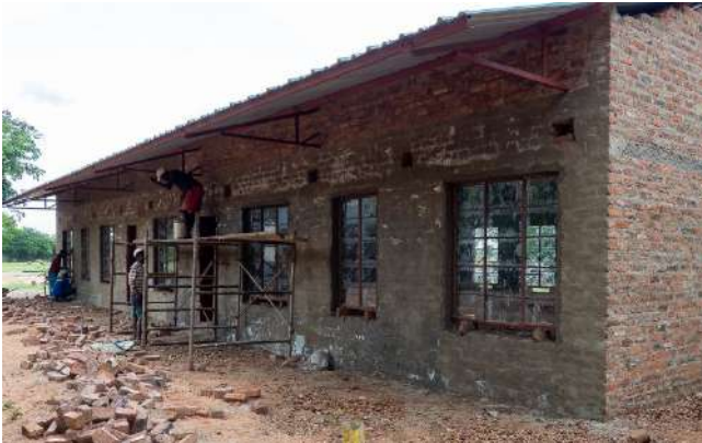
Completing the 5 th classroom block
