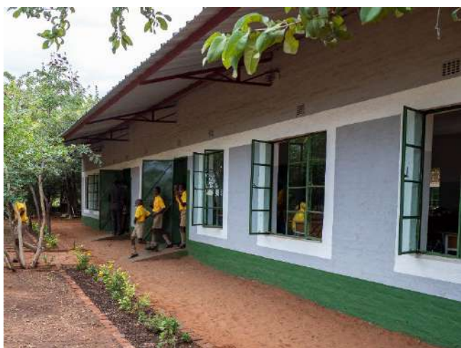
The new school has two double classroom blocks
