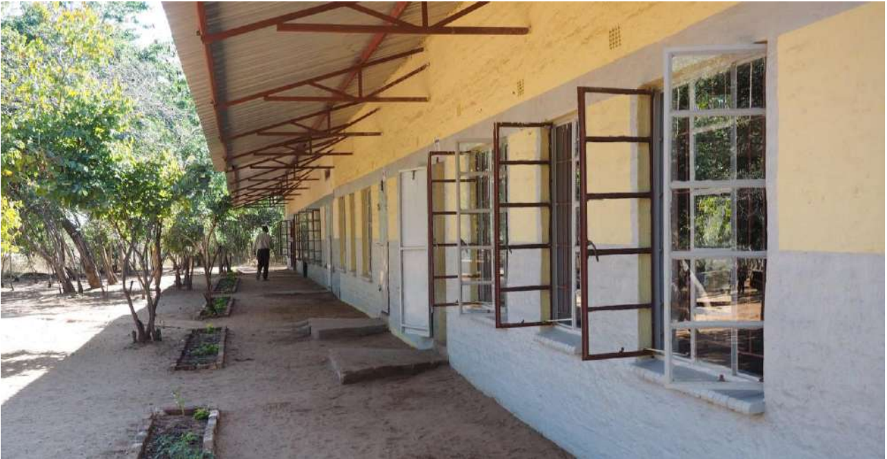
Classroom Blocks I and II now joined by a library/office
