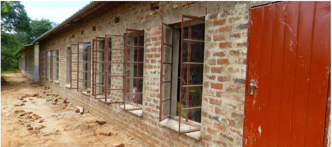
Second classroom block, already in use for Grade 1
