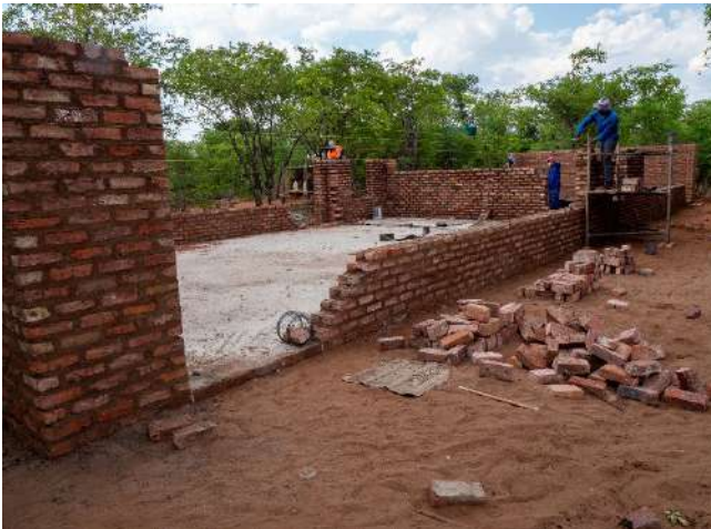
Vocational blocks under construction
